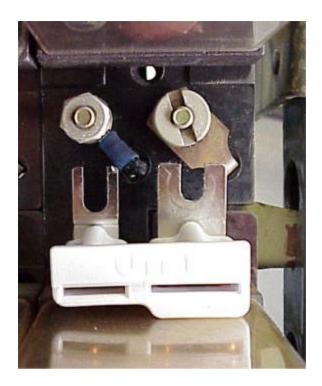
The following is a picture of a connection block attached to a B1 relay.
